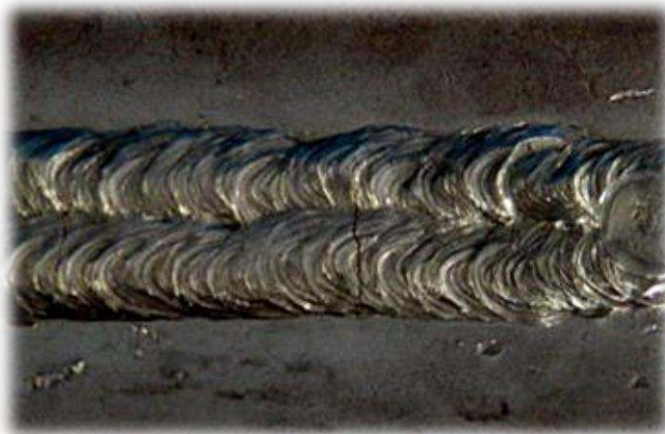
Figure (II.2) Les fissures transversales.
