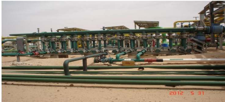
Figure III.13 : Manifold [14] .
