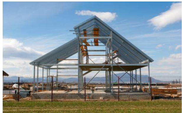
Figure 16: Structure en acier. Source: www.le-guide-de-la-maison.com
