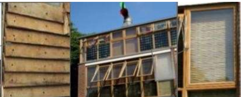
Figure 26: la protection solaire mobile
