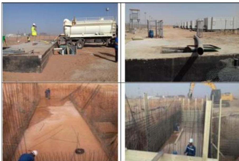
Figure II.24 : Fosse septique BDV 58 cabines
